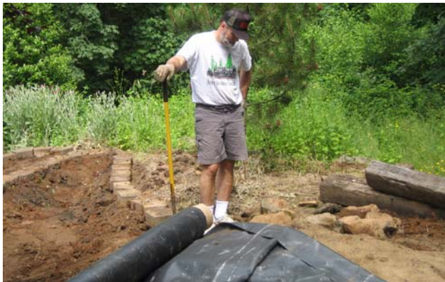
Jeff Lange excavates for a pond
