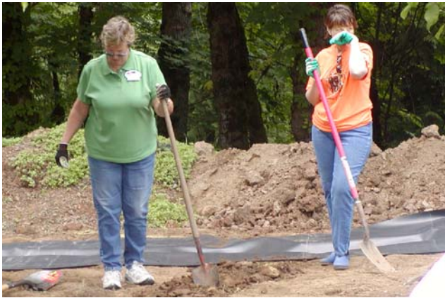
Penny Walker and Barbara Clark excavate for a track bed.
