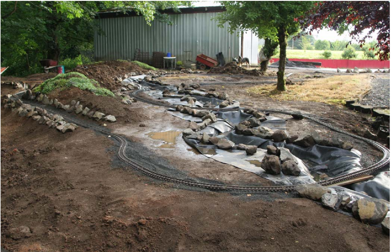
Track is set in place. Much landscaping in the future.
