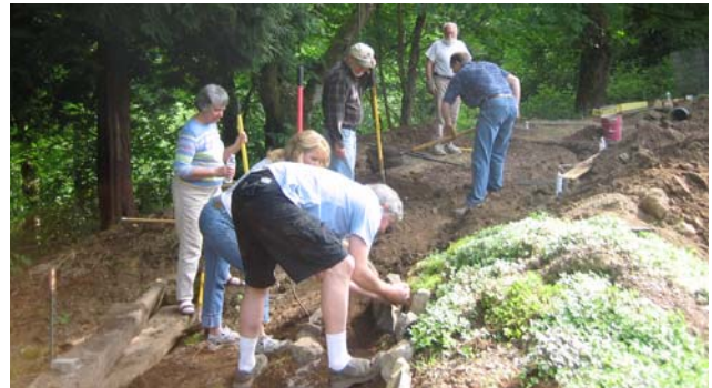
Sculpting mountains, and trenching the Georgetown Loop"
