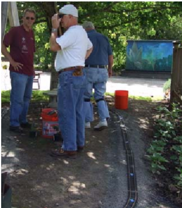
Taking a break from installing track on the ground.
