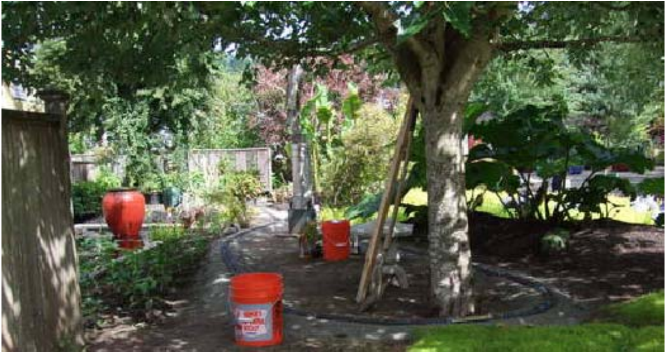
The work area
