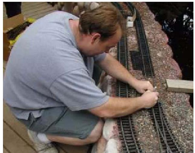
We did not expect cutting and bending stainless steel rail to be so difficult. Dave Linn brought an air grinder to cut rail. It was still a lot of work. Jeff brought a rail bender, but Gary preferred the handle on our rail bender. I also observed Jeff bend an as-
