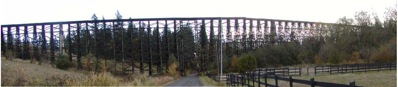
One of the highest and longest trestles in Oregon. This Portland & Western/Willamette & Pacific Railroad trestle crosses over NW Dick Road about two miles north of Hillsboro, Oregon. This trestle is approximately 150 feet tall and 1,200 feet long.
